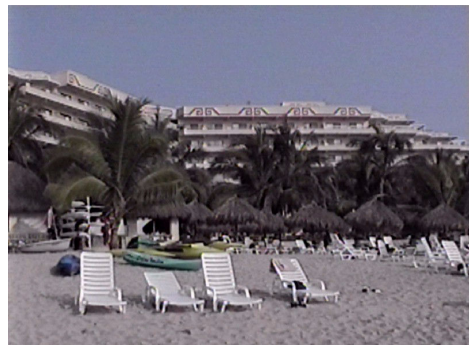
The new Tikal Tower at Paradise Village
